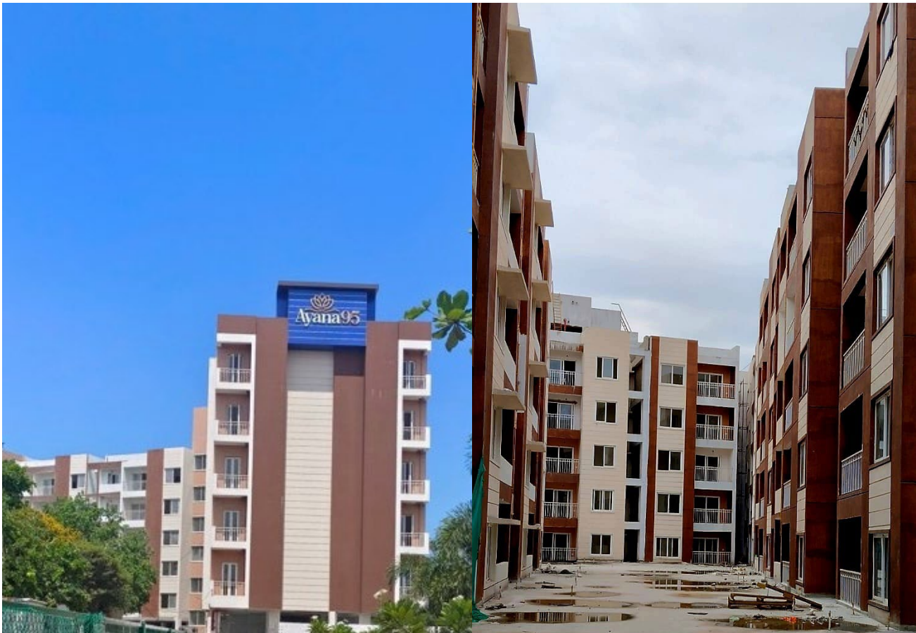
DaaS delivered project in Chennai
